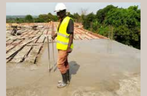
Well-laid Maxpans on the shutter before concreting
