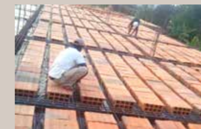
Well-laid Maxpans on the shutter before concreting
