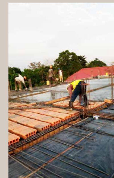
Well-laid Maxpans on the shutter before concreting
