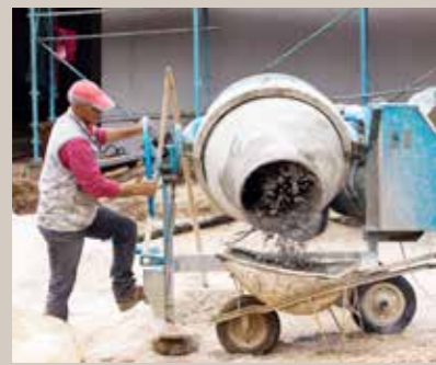
Aggregate used in concrete mixing
